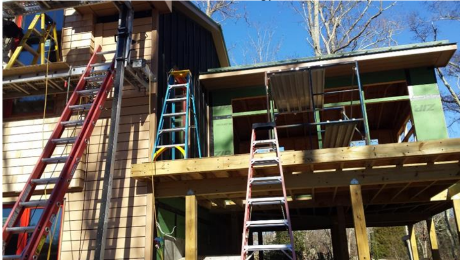
(Above is the passive house under construction)
