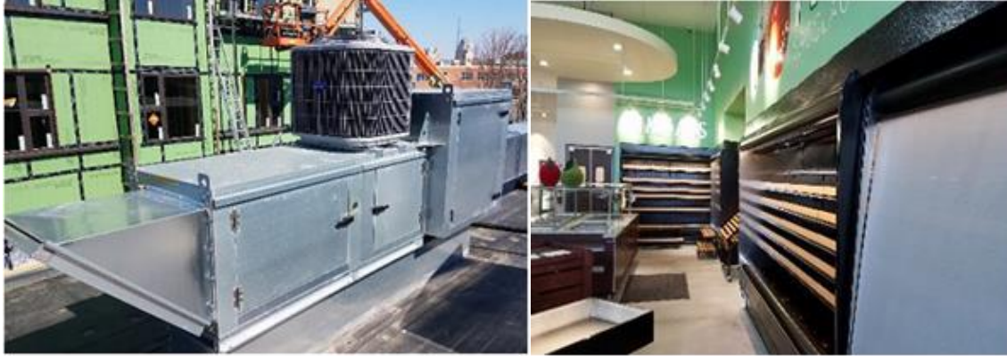
CaptiveAire kitchen exhaust hoods (left) and Night Covers (right) at the Urban Greens Co-Op, Providence
