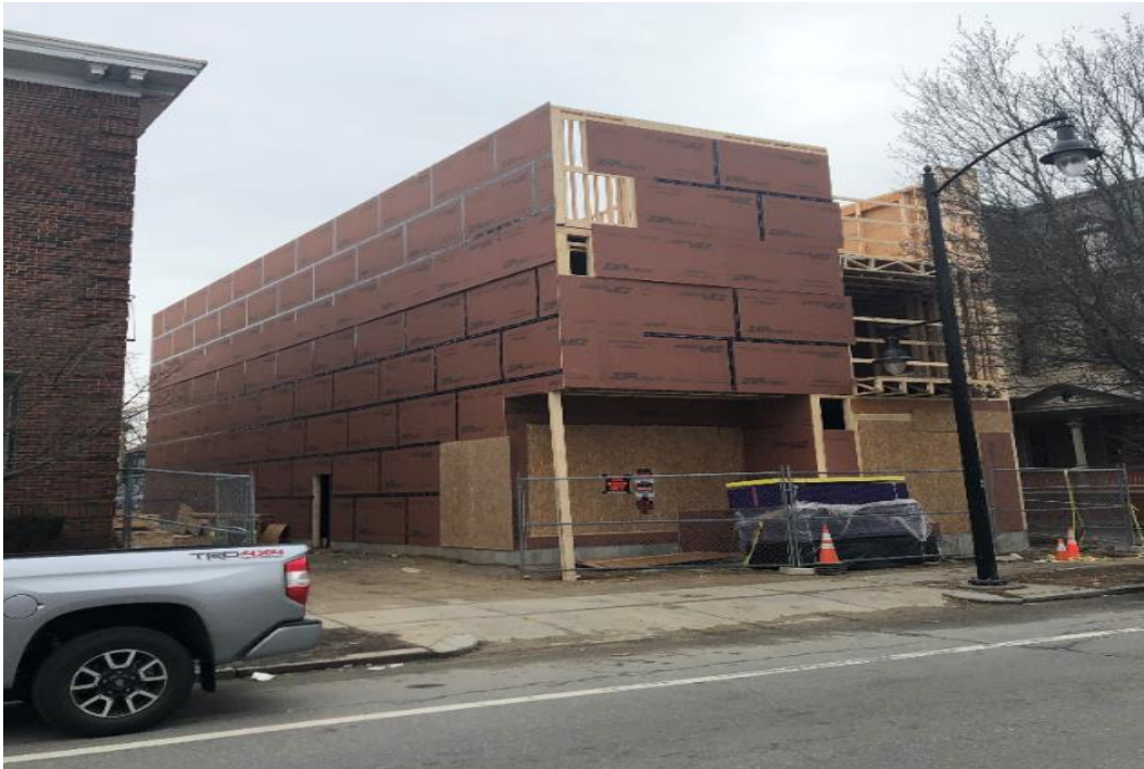
Pictured above: Westminster Street Multifamily Passive House, Under Construction
