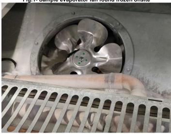
Fig.1- Sample evaporator fan found frozen onsite
