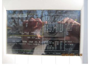
Photo 2-7 above shows that the suction head of the CO<sub>2</sub>-based system is at 413.9 psig. The evaluators used the temperature-pressure (PT) chart for R-744 (CO<sub>2</sub>) and determined that the saturated condensing temperature (SCT) at 413.9 psig is  $21.2^{\circ}$ F.
