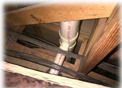
Plumbing/Wire Penetrations (before)
